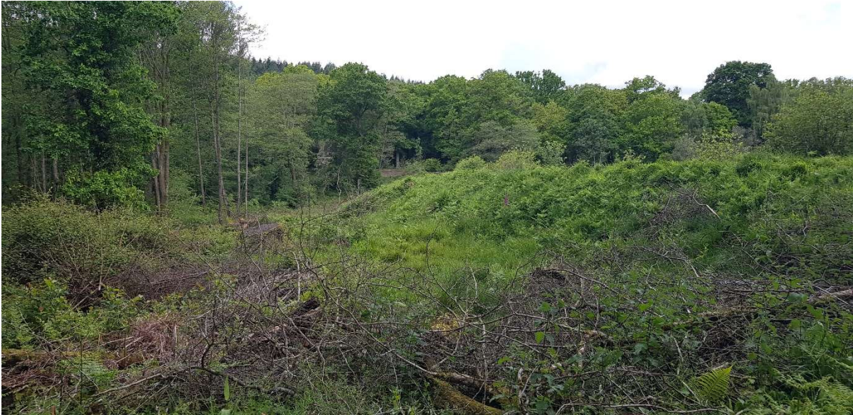
Photograph 1: General view of embankment
