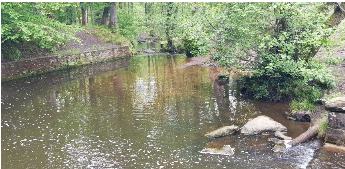
Photograph 14: Spillway stilling basin
