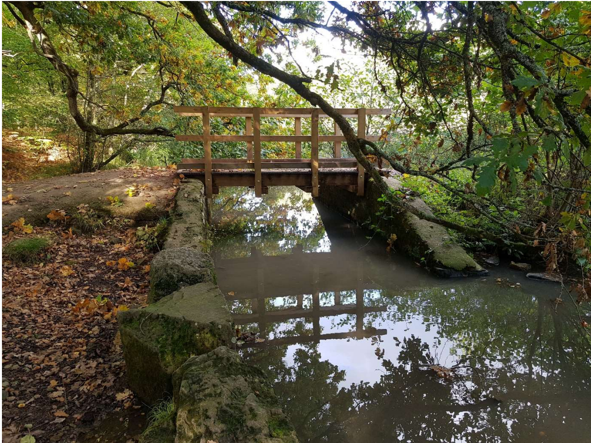
Photograph 19: Channel through causeway embankment joining the north and south sides of the pond
