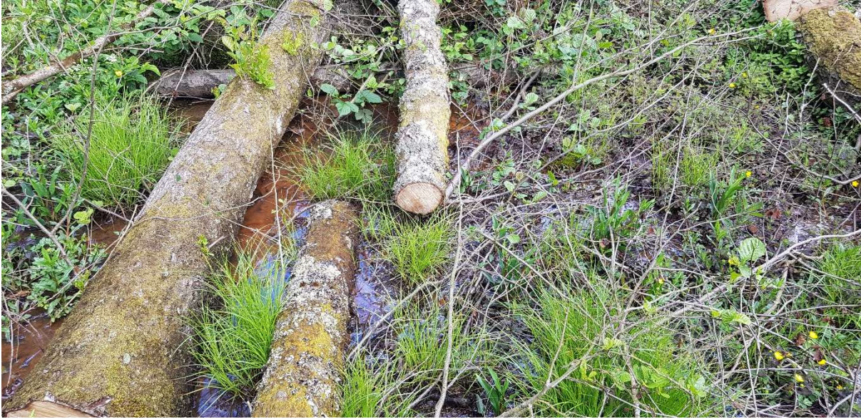
Photograph 7: Wet area downstream of embankment toe
